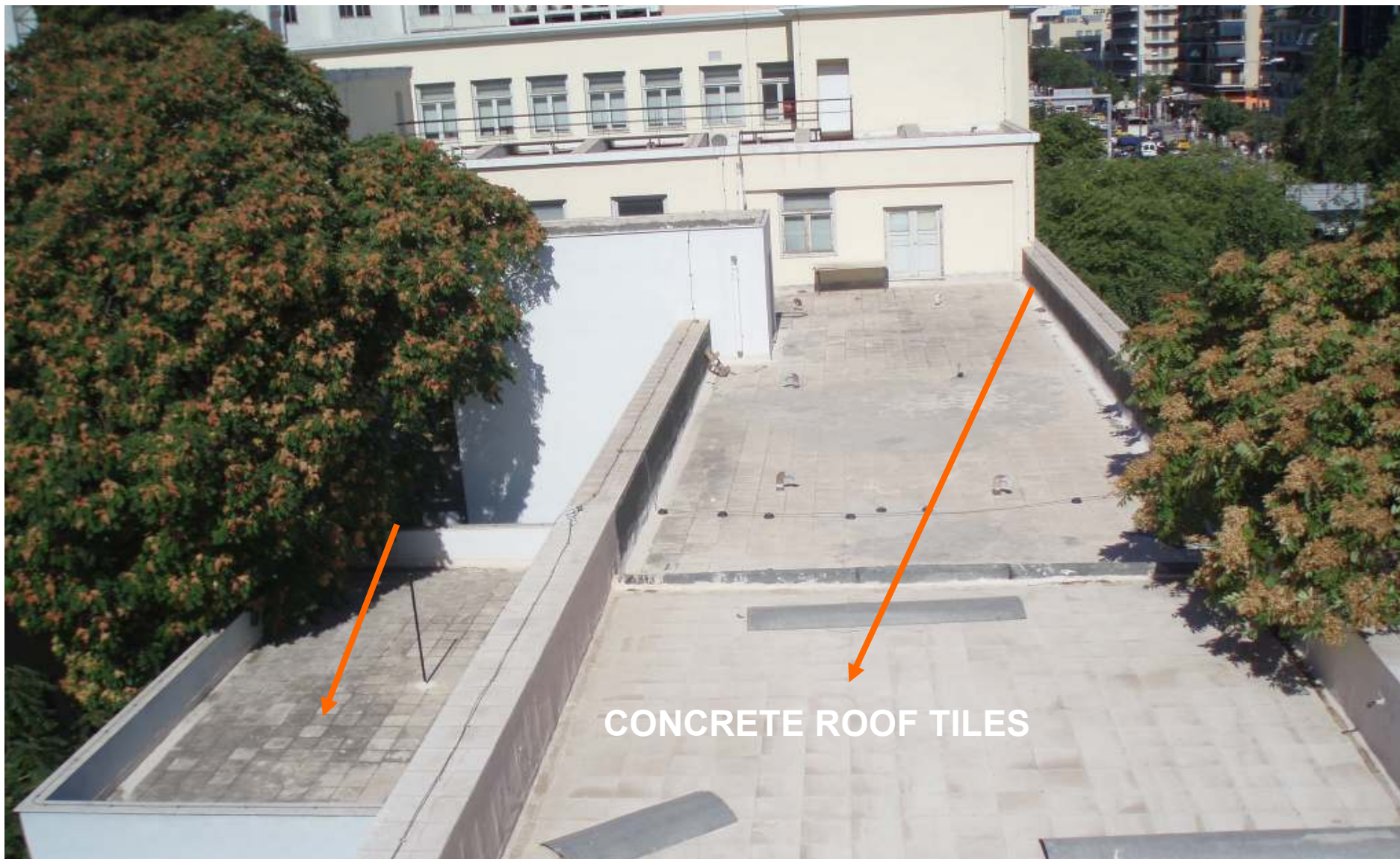
PREFECTURE OF ATHENS- DEPARTMENT OF SOCIAL PROVIDENCE ROOF BASED ON CORRODED CONCRETE ROOF TILES APP. 600 m 2
